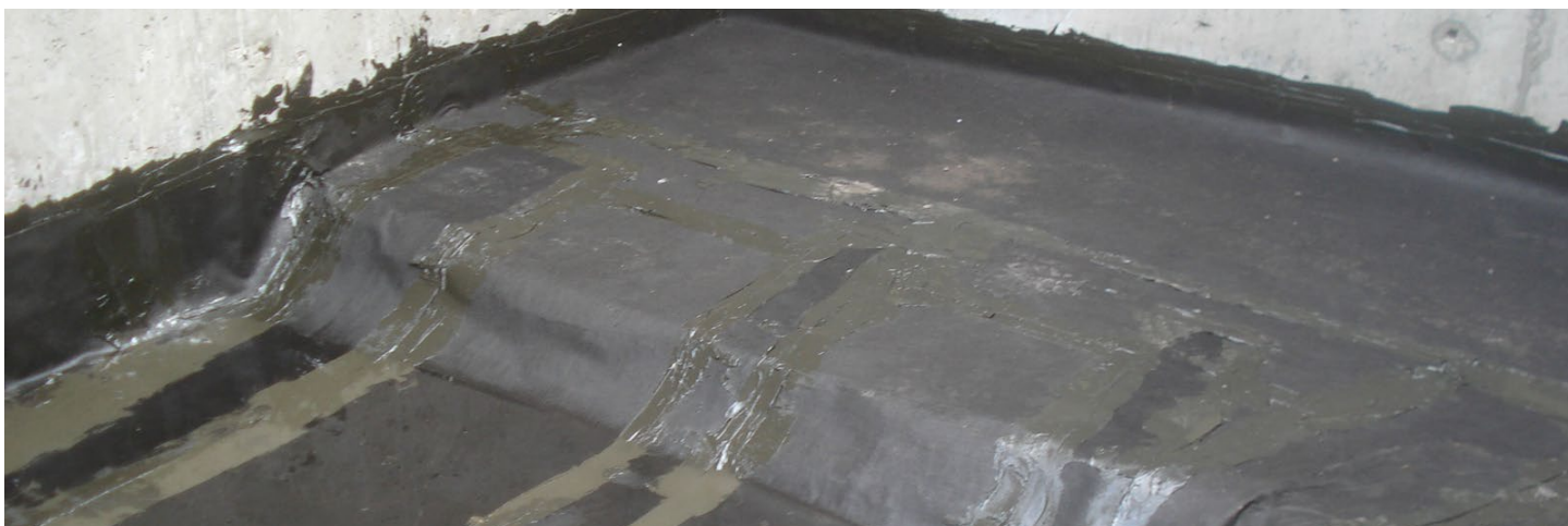
PRECON sheeting was applied before concrete was poured to protect the basement floors from underground seepage.
